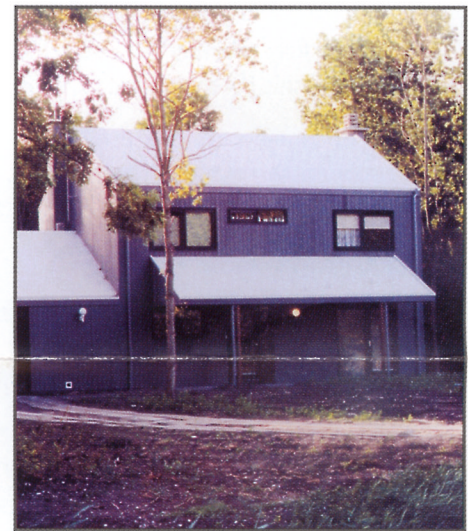
Eco Housing project in Zwolle.
