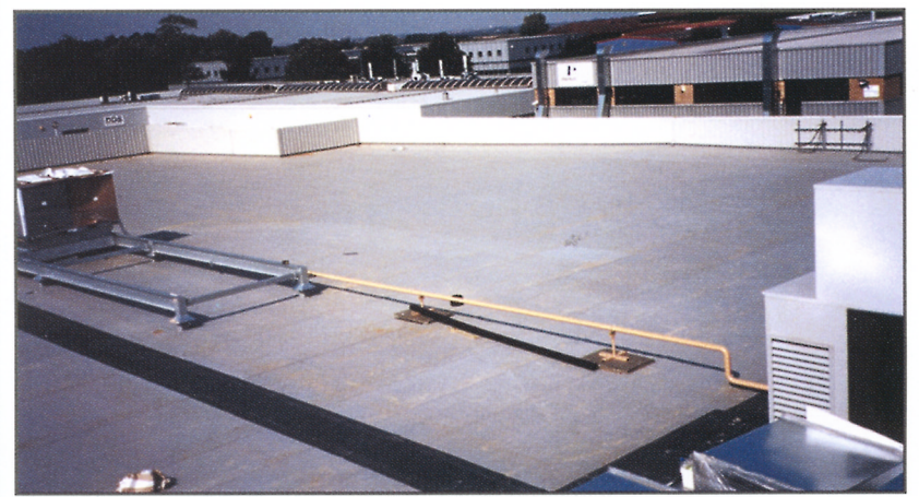
Tesco in Bar Hill - 15.000 m 2 mechanically attached system
