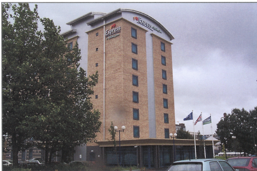
Holiday Inn in Lichfield - mechanically attached system + profile
